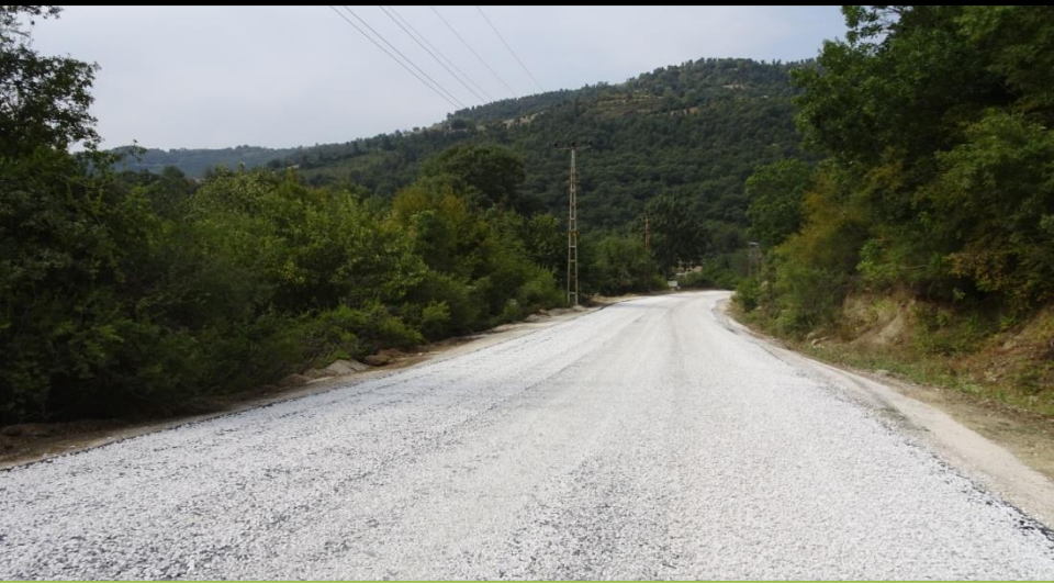
HASANBEYLİ KARAYİĞİTLİ 2. KAT ASFALT
